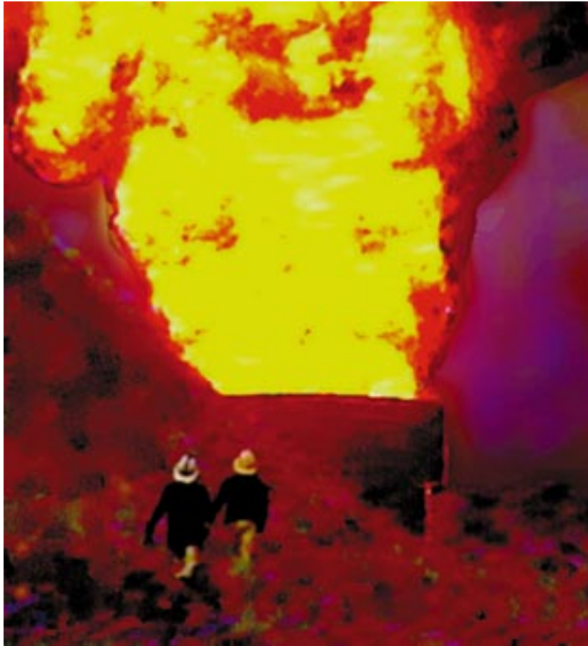
Figure 2. Flames over 120 m high burning above one of the Summit Tunnel's vent shafts in December 1984 (Yorkshire Television news footage).
